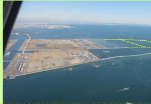
Tokyo Bay Offshore Final Landfill Site (2009.1.13) Left: Current Operating Site (314ha), Right: Construction of New Site (184ha)
