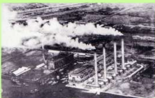
Fukagawa Incineration Plant (1933), Capacity: 940t/day
